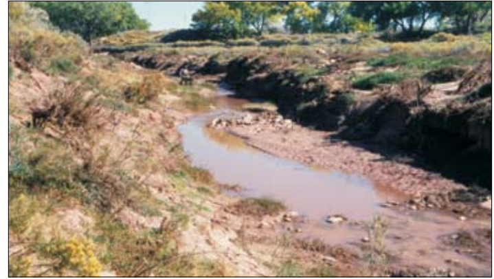
Channel response to the rock baffle at Hubbell by October 1999. (Photos courtesy of Bill Zeedyk.)
